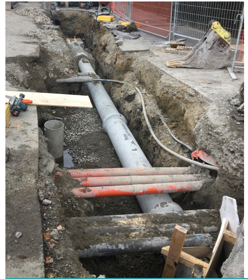
Above: Example of new drainage laid at the intersection of Barbadoes Street / Warrington Street.
